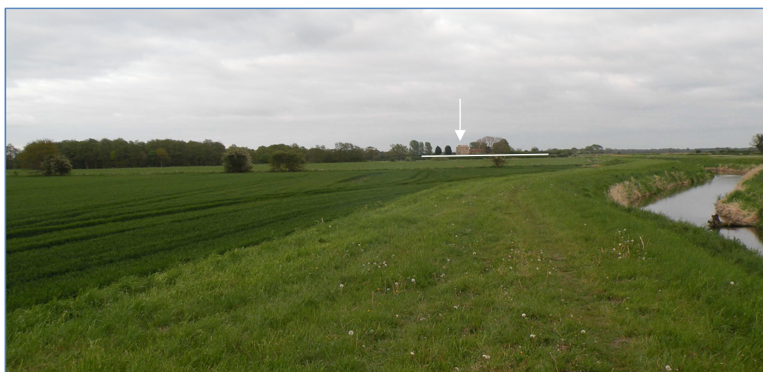
Photograph 2 View from PAA towards Pentney Priory. The scheduled boundary is highlighted in white and the gatehouse is arrowed
