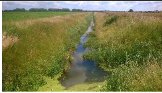
21 TN14 'Forty foot' drain looking west
