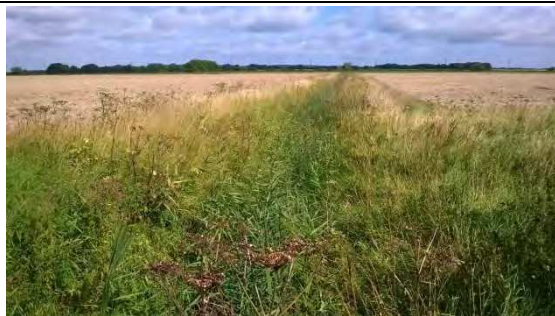
56 View of drain
