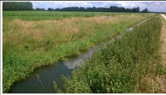
41 TN32 Forty-foot drain
